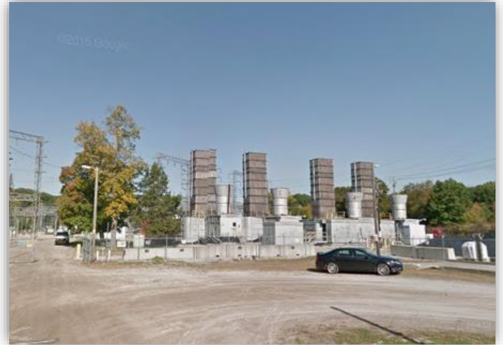
Photo Credits: Google Earth
