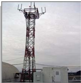
A 1-kW fuel cell system has been providing power for this FAA radio tower near Chicago for more than three years. (Photo courtesy of ReliOn)
