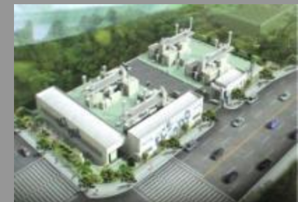
11.2 MW power plant
