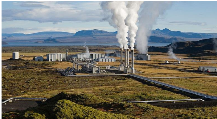
Geothermal Power Plant in Iceland. http://en.wikipedia.org/wiki/Geothermal_energy
