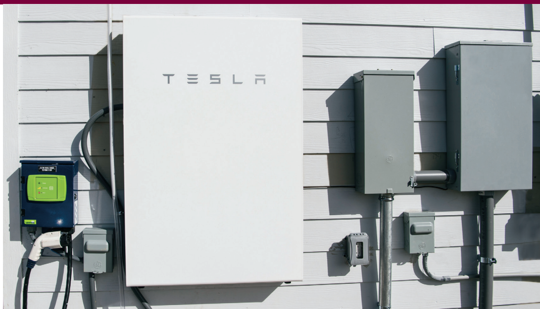
Lithium-ion battery installed on the exterior of a home.
