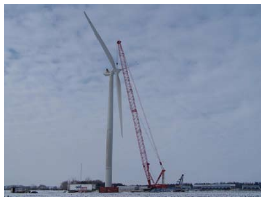
Construction of the 1.65 MW wind turbine at the Morris research center.
