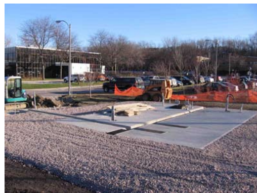
Demonstration site at the Vermont Department of Public Works in December 2005. This picture shows the platform ready for equipment to be installed.
