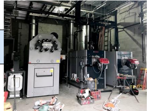
UNH Biomass Boilers & Precision Dried Chips Storage
