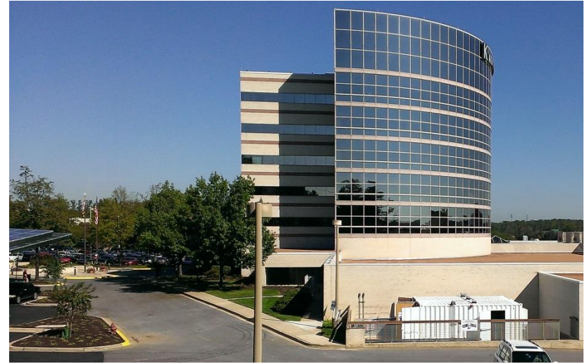
Konterra Headquarters Laurel, MD – 500kW
