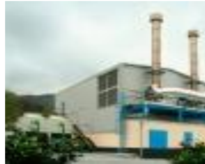
Gas Turbine CHP Plant
