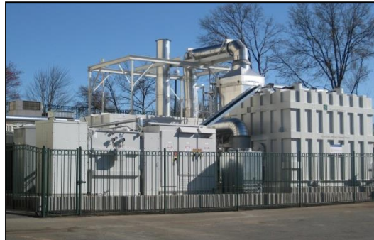
1.4 MW Steam CHP for campus energy system at University in CT
