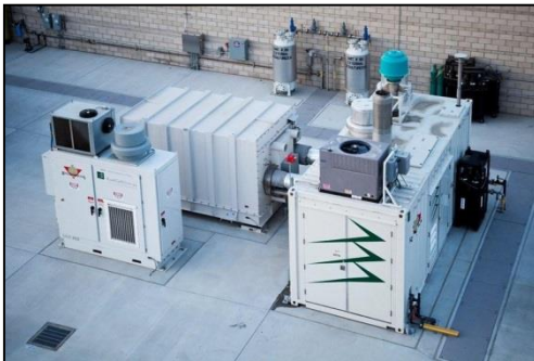
300 kW Hot Water CHP for Onion Waste digester in California
