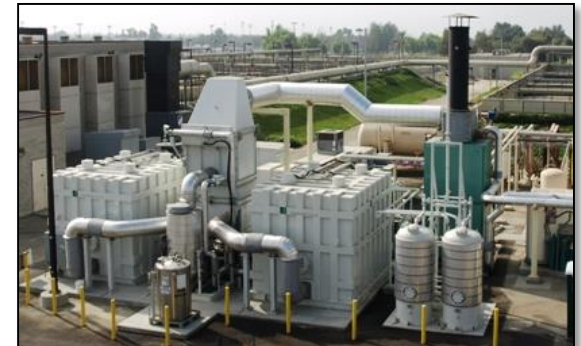
2.8 MW Hot Water CHP Waste Water Digester Plant in California
