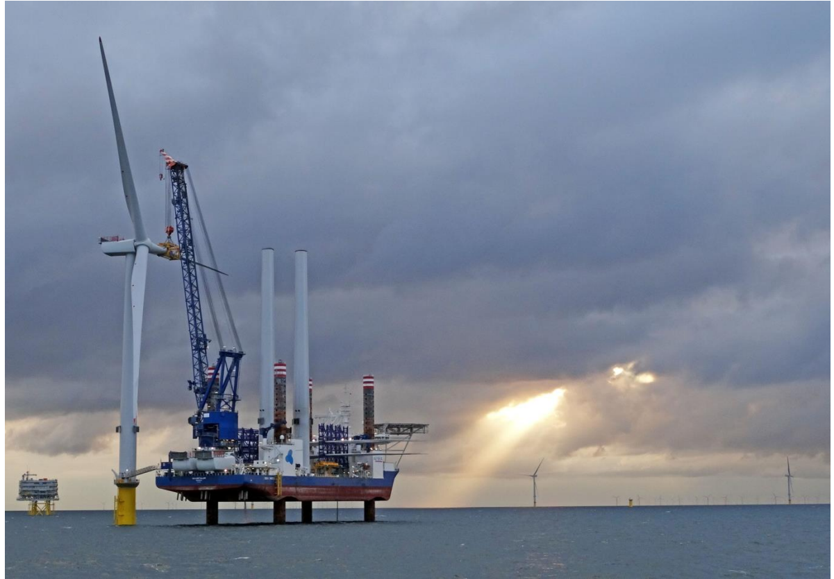
MHI Vestas V164-8.0MW turbines being installed at the Burbo Bank Extension
