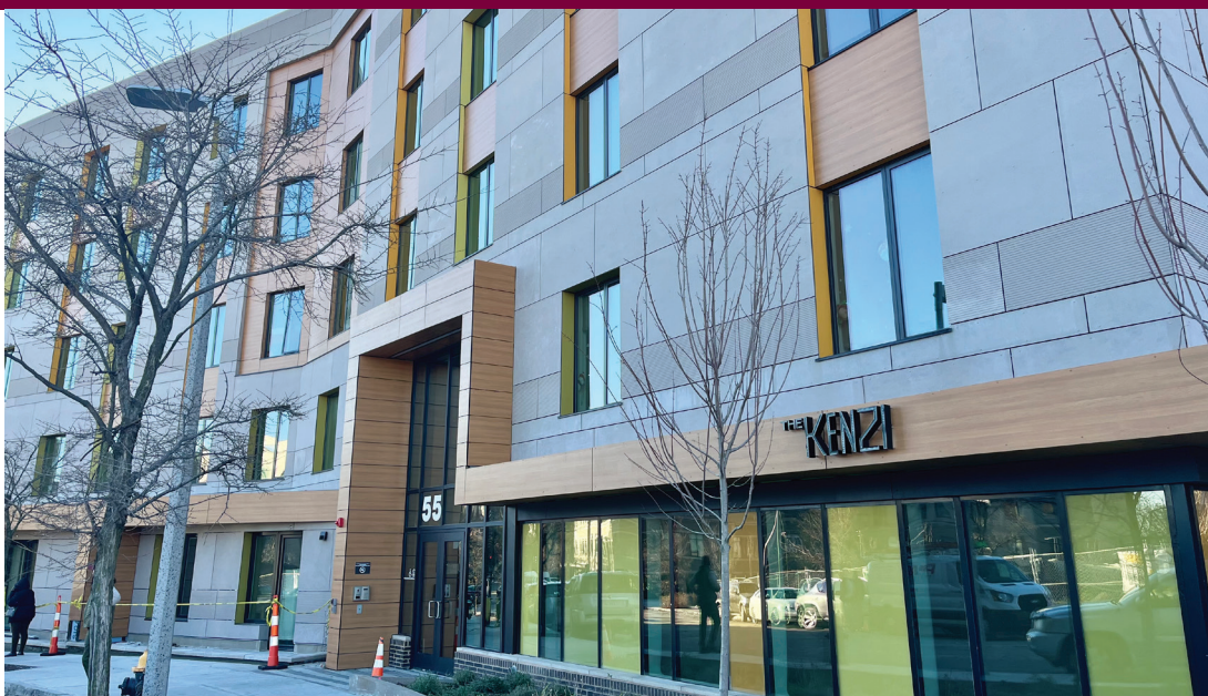
The Kenzi Apartments in Boston, MA is equipped with solar and battery energy storage to power an on-site community resilience hub.
