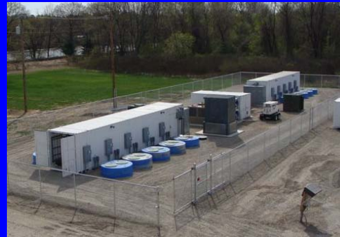
2 x 1MW / 15 min Flywheels in NE-ISO
