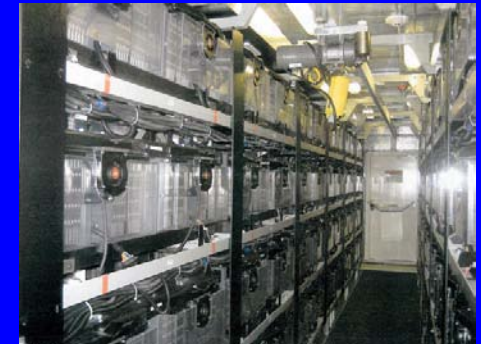
4 x 1MW / 15min Li-Ion in PJM. CA-ISO
