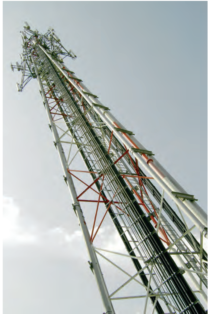
More than 6,000 fuel cell systems have been installed at cell phone towers across the United States. © ReliOn
