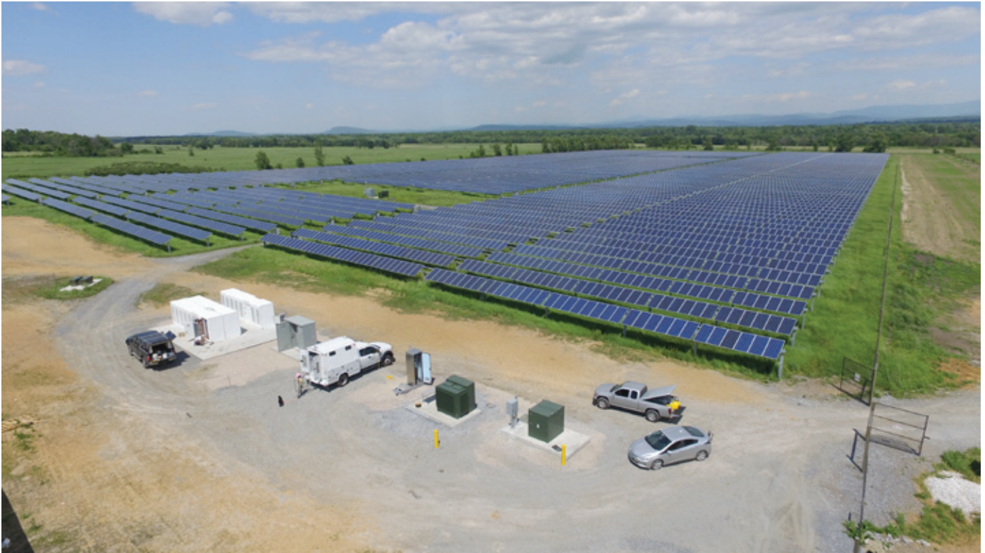
Green Mountain Power's Pantan, VT solar+storage project combines 5 MW of solar PV with 4 MWh of battery storage. The utility is using this project to pilot its “resilience zones” concept. By adding switches to the existing distribution grid circuit, GMP can provide backup power from the solar and batteries to surrounding homes and businesses in case of a grid outage.
