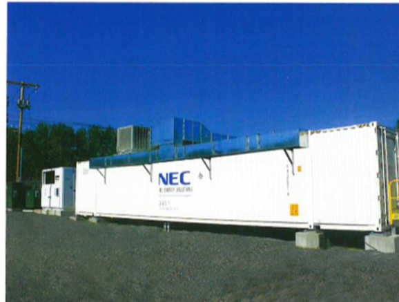
2MW energy storage system built by NEC for Sterling Municipal Light Department in Sterling, Massachusetts.
