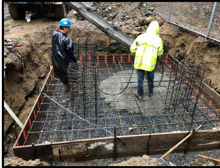
1 or 2 Battery Container Foundations
