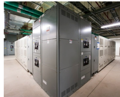
1.08 MVA Grid Simulator
