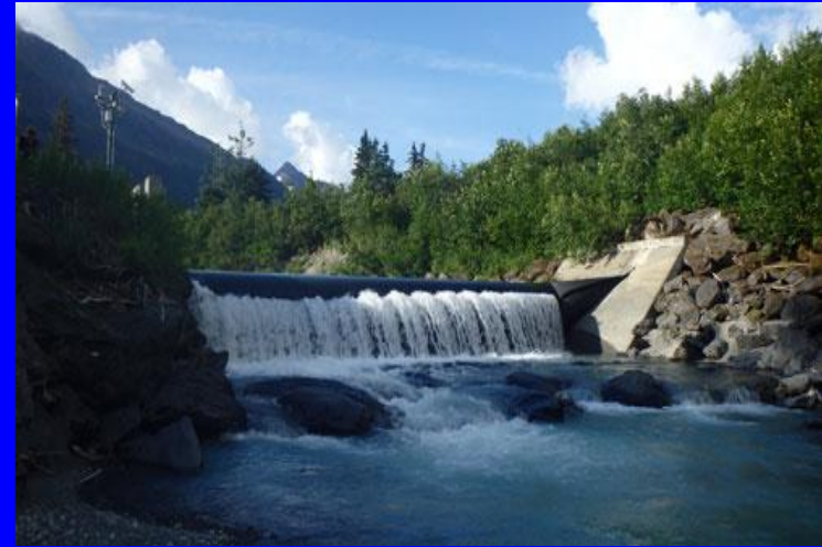
6MW Run of River Hydro Power
