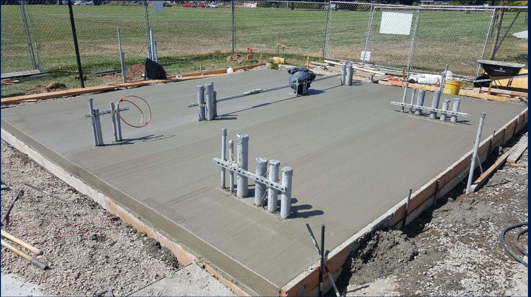
Main BESS pad poured – 12" thick
