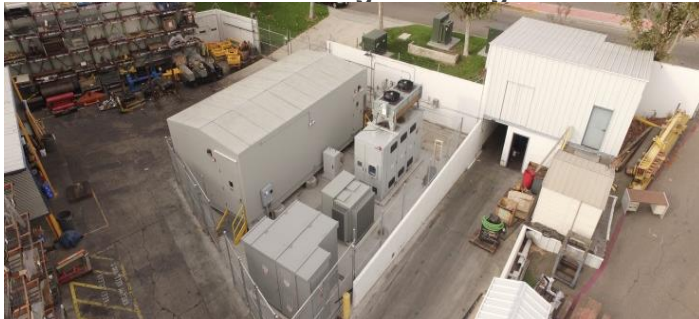
Custom enclosure GSS ® grid storage solution
