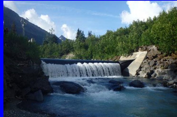
6MW Run of River Hydro + 2MW Diesel
