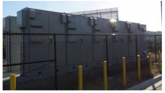
125kw 2.4 hour system supporting a 30kw PV.
