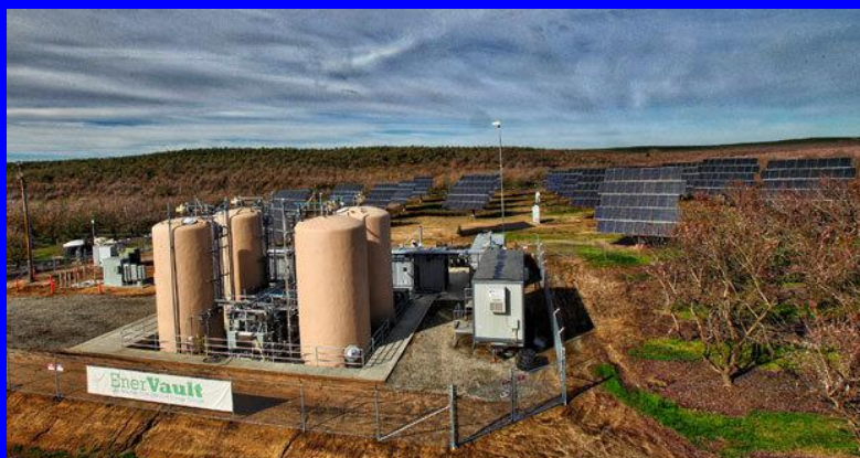
Installation of Tanks at Turlock
