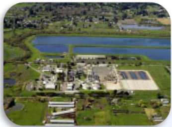
Waste Water Treatment Plant
