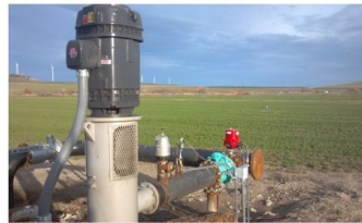
200 HP MOTOR WITH VERTICAL LINE SHAFT PUMP – 8” PIPE, AQUIFER LEVEL 520 FEET BELOW LAND SURFACE.
