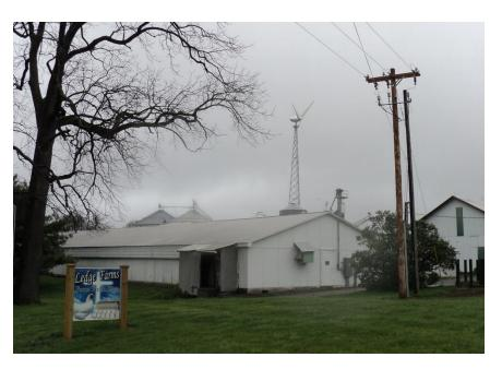
50 kW Produces 100 to 160,000 kWh Cost \$350,000
