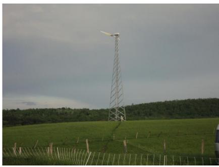
11 kW - Produces 16 to 30,000 kWh - Cost: \$125,000
