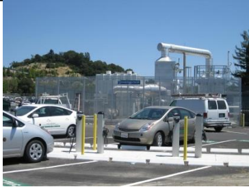
1.4 MW plant at a municipal building
