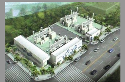
11.2 MW power plant
