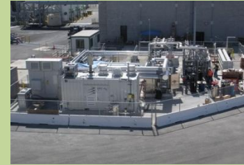
Renewable biogas fueled DFC300-H2 in CA providing hydrogen for vehicle fueling under DOE demonstration program
