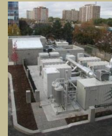
Renewable biogas fueled DFC300-H2 in CA providing hydrogen for vehicle fueling under DOE demonstration program
