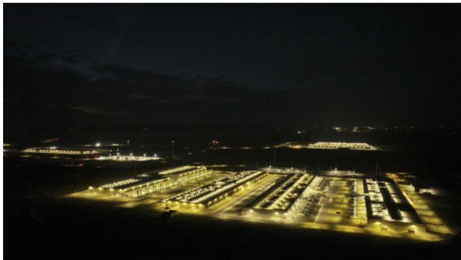
Amazon Web Services Data Center in Boardman Oregon, August 2024. (AP/Jenny Kane)
