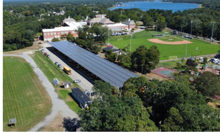
Nauset Regional Middle School Canopy & BESS
