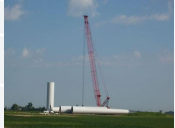
Construction of Port Alma Wind Farm
