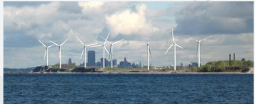
Steel Winds Project on the Buffalo Waterfront
