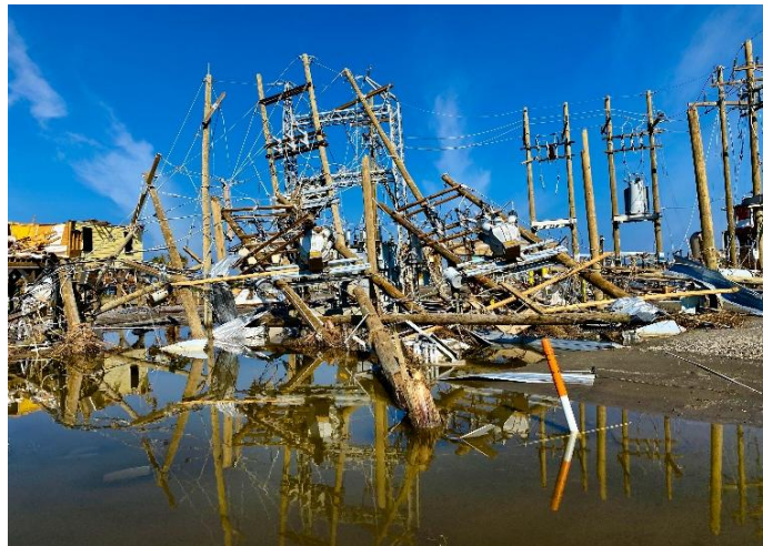
Damaged energy infrastructure in Grand Isle, Louisiana following Hurricane Ida. Credit: Ed Lallo / iStock.
