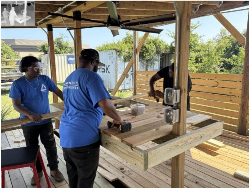
Groundwork New Orleans staff and participants construct the outdoor classroom and resilience shelter at the NET Charter High School: Gentilly. This space, which is powered by the Queen Bee, serves as a class workspace, cooling area, and charging station. In the event the Queen Bee has to be delayed, the site has separate solar+storage to run the outside loads. (Credit: Groundwork New Orleans)
