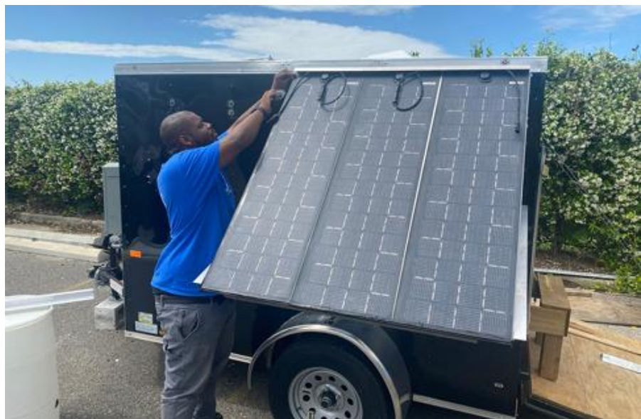
Groundwork New Orleans staff construct the first Bee - a mobile solar+storage trailer. (Credit: Groundwork New Orleans)
