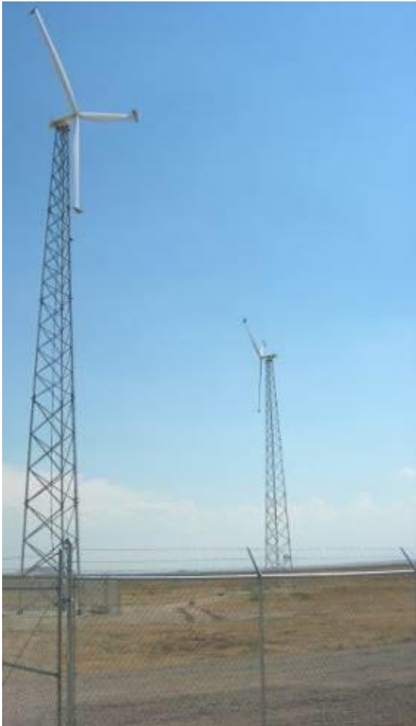
Entegri Wind Turbines
