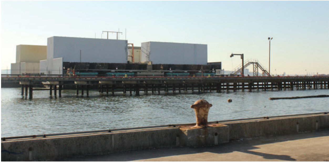
Eastern Generation's Narrows peaker plant in Brooklyn. PHOTO: UPROSE
