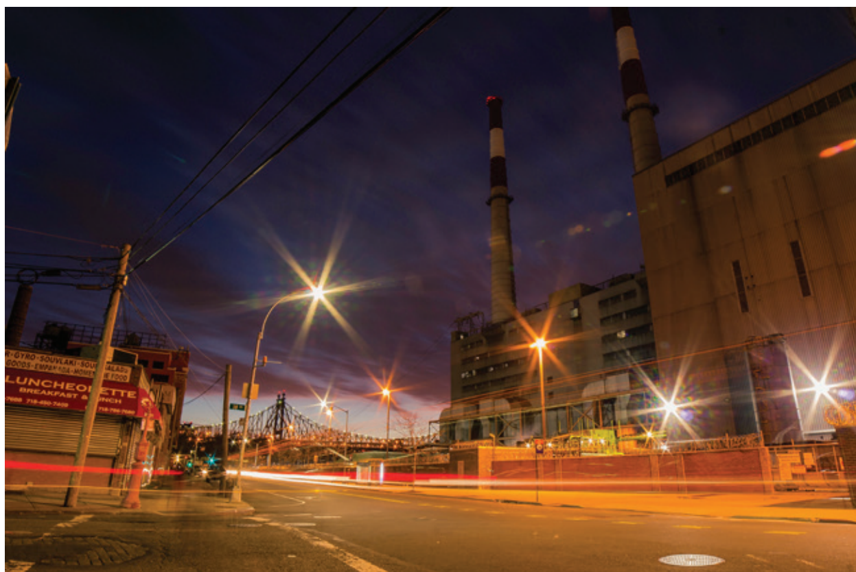
Rise Light & Power’s Ravenswood Generating Station in Queens. PHOTO: SEBASTIAN BAEZ/UPROSE
