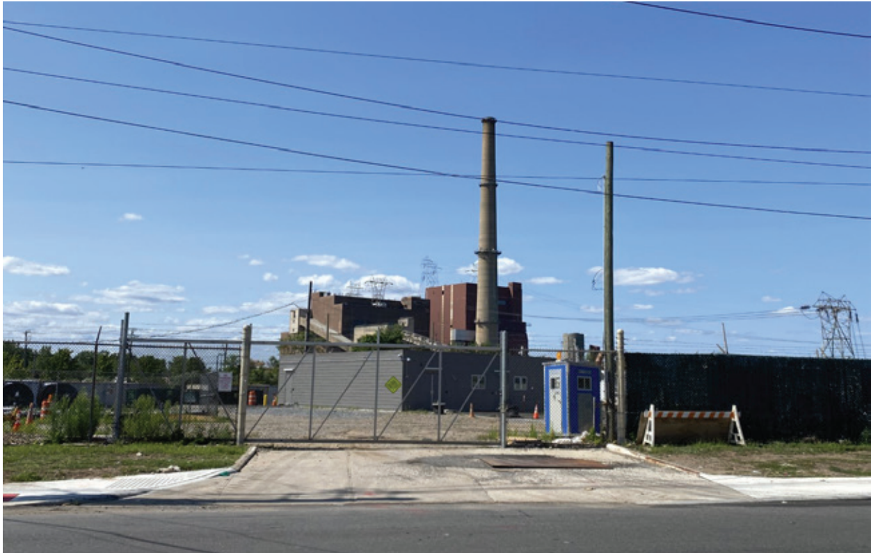
NRG's Arthur Kill peaker plant on Staten Island. PHOTO: JUSTIN WOOD/NYLPI
