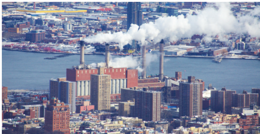
ConEd's East River Generating Station in Manhattan.
