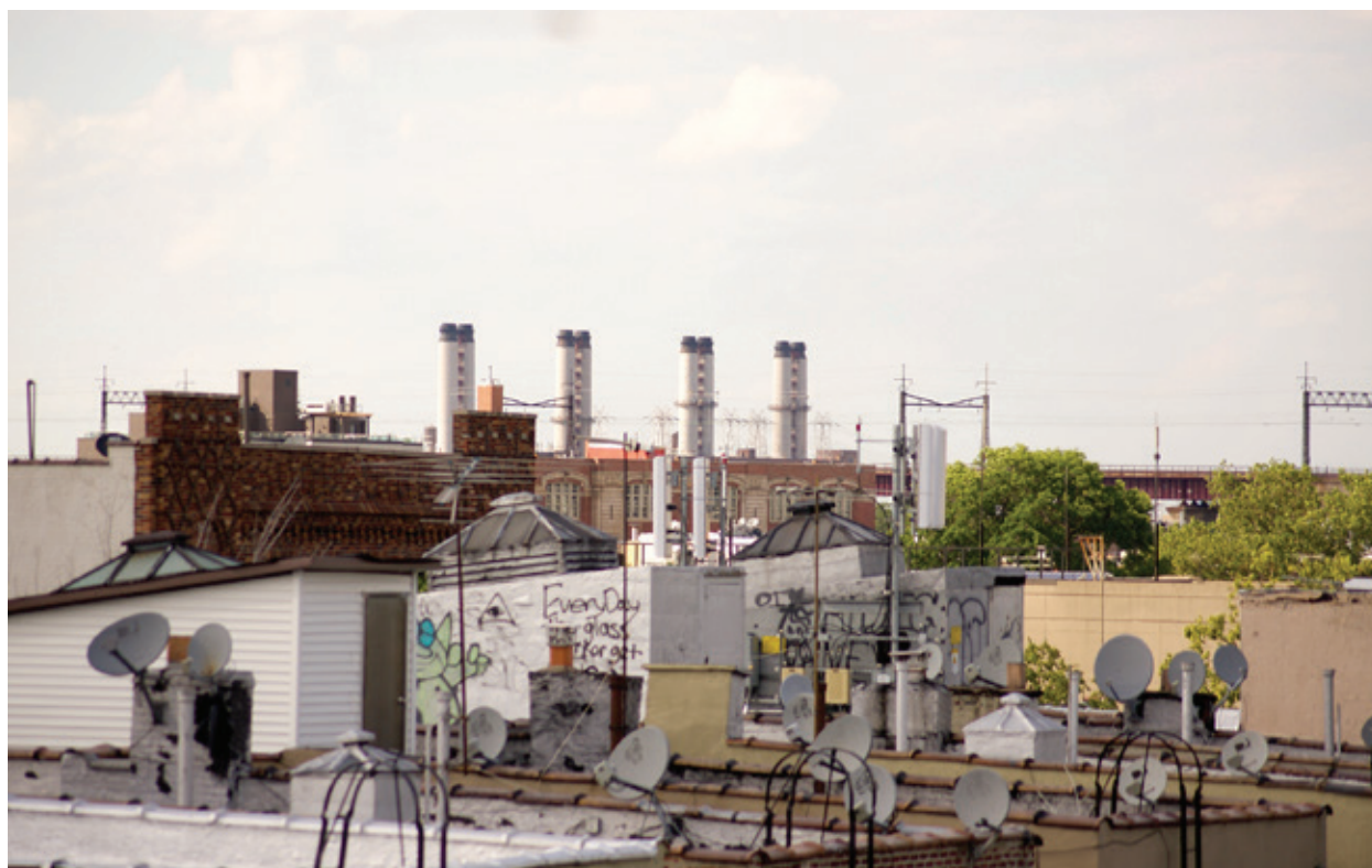
Eastern Generation's Astoria Steam Turbine Generating Station in Queens. PHOTO: SEBASTIAN BAEZ/UPROSE
