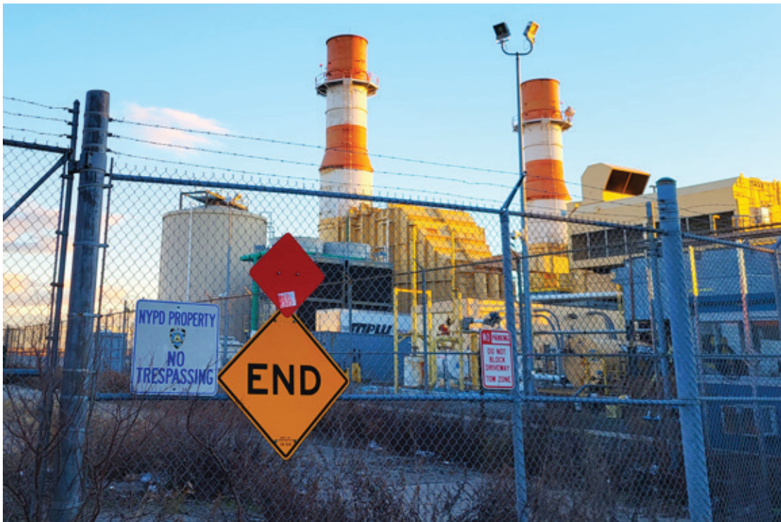
Hell Gate peaker plant in the South Bronx. PHOTO: EMILY SWANSON
