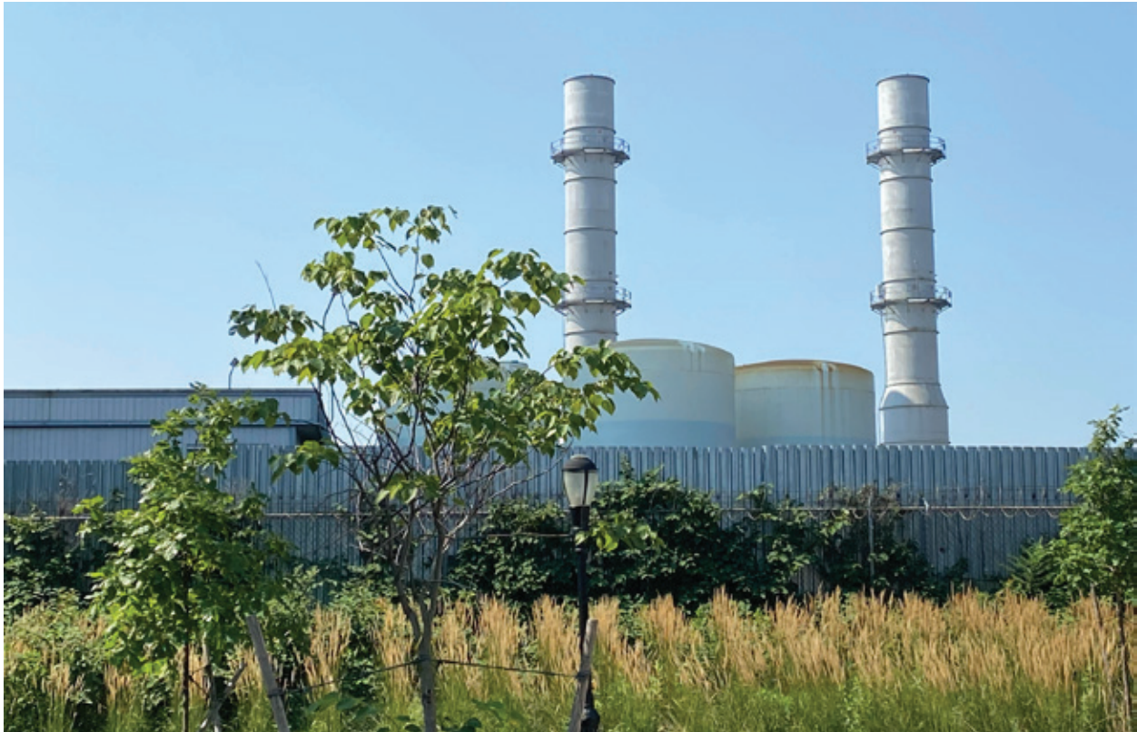
NYPA's Vernon Boulevard peaker plant in Queens. PHOTO: UPROSE
