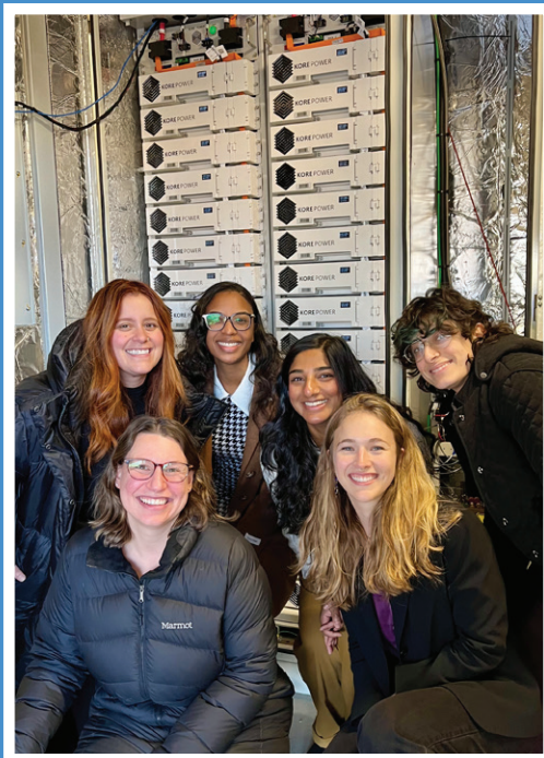
Clean Energy Group staff tour the battery storage unit at the Kenzi Apartments in Roxbury, MA in December 2024. Clean Energy Group's Technical Assistance Fund supported a resilient solar+storage system at this low-income senior housing building. Photo: Clean Energy Group.
