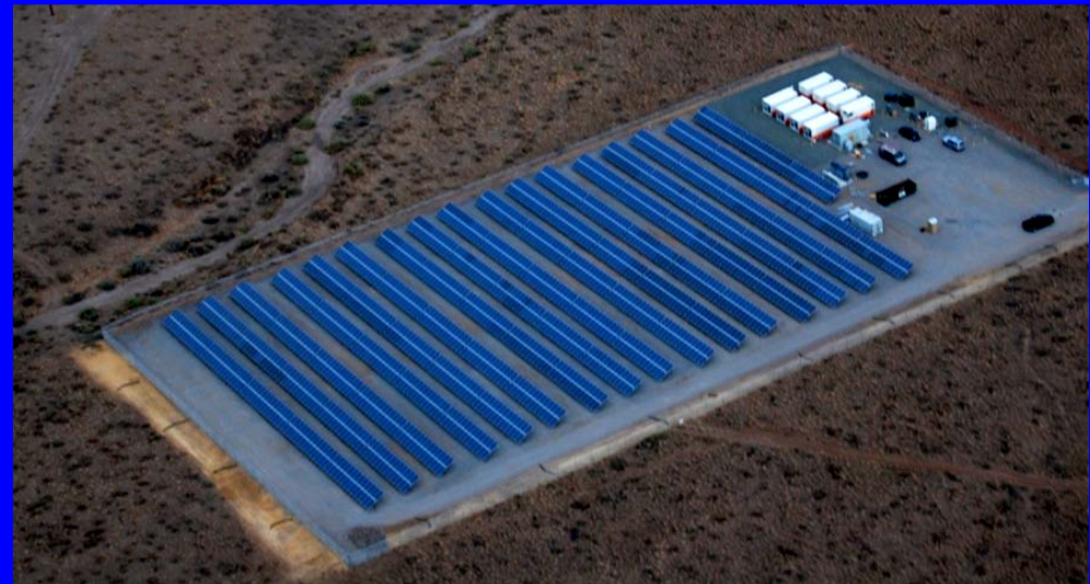
Commissioned Sep. 24, 2011 Integrator: Ecoul
