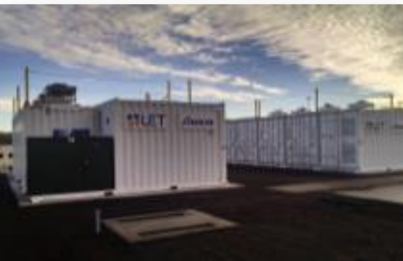
Avista/UniEnergy 1 MW/4 MWh System installation February 2015, commissioned in June.
